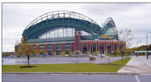
(Above) Uni-Systems utilized actuators from Nook Industries to solve a persistent water problem at Miller Park, the new home stadium of the Milwaukee Brewers.
